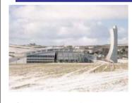
Combust waste under controlled conditions, to reduce its volume and hazardous nature, and to generate electricity and/or heat
